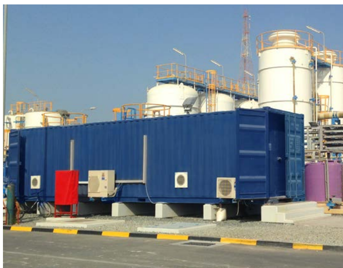
Scotmas Bravo MX duty / standby system in 40" container, installed in Qatar.
